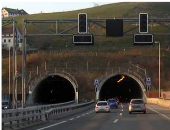
Portal Tunnel Uznaberg
